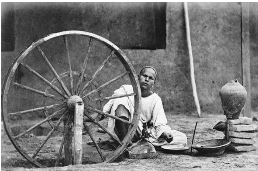
Figure 14. Silk production. Unwinding silk on a spool. Turkestanskii Al'bom (1872). Reproduced from Library of Congress.
